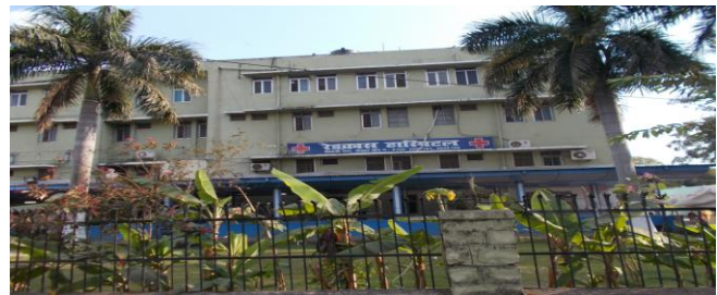
Red Cross Hospital, Bhopal
